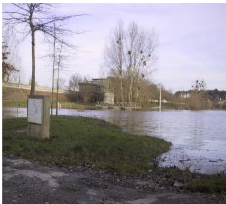
Station d'eau potable Chalonnnes-sur-Loire
